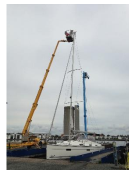
Reparation i mastetoppen
